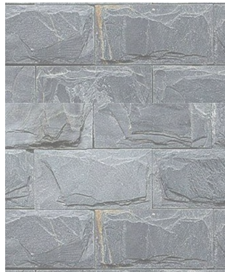
6. MASONRY BASE ELEMENTS
