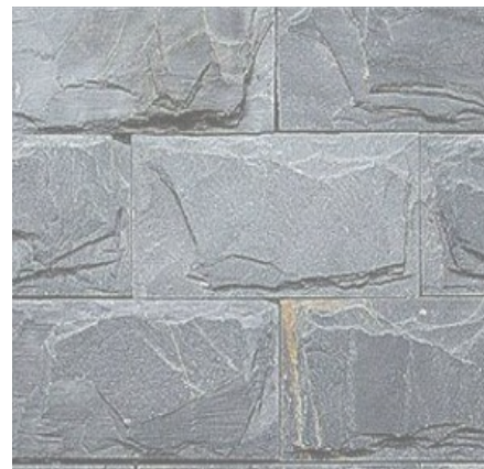
6. MASONRY BASE ELEMENTS
